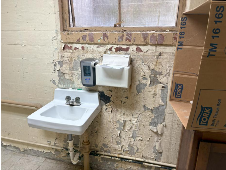
Pictured, basement unused bathroom, failing paint.
