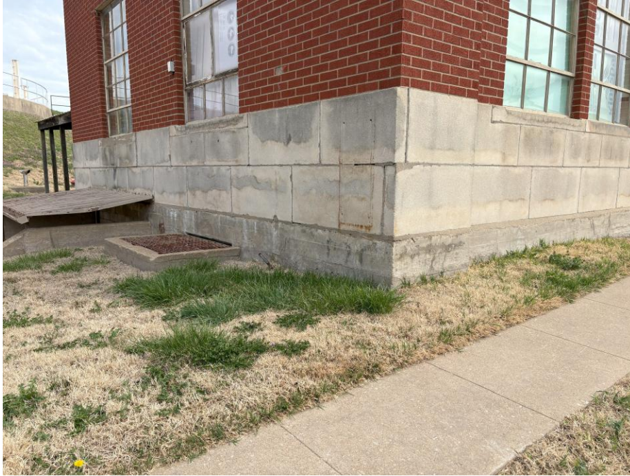
Pictured, Southwest corner, shifting masonry, spalling and missing mortar joints.
