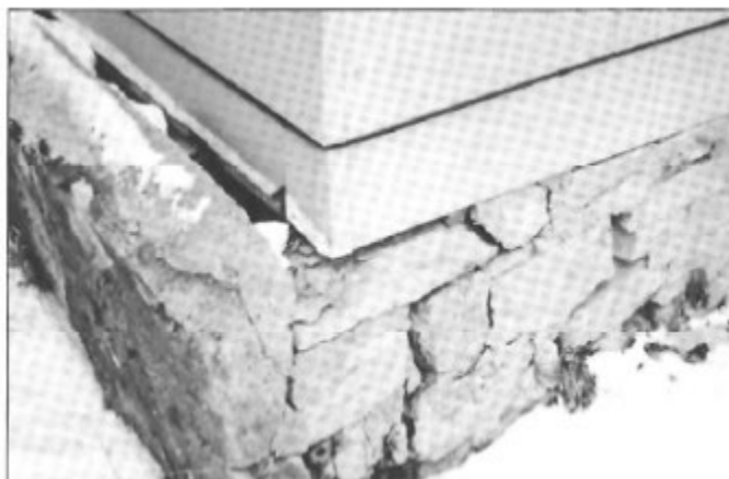
Commentary Figure 304.5—Major Damage to a Foundation Wall
